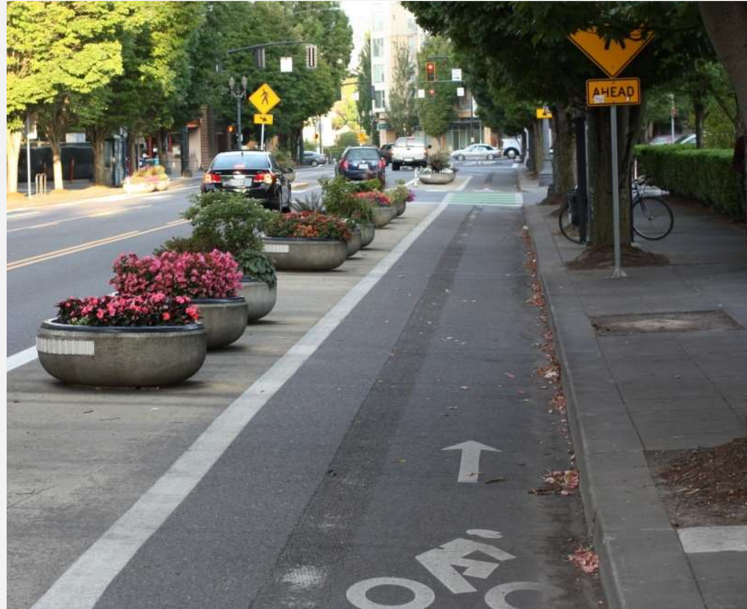
NE MULTNOMAH STREET LOOKING WEST
