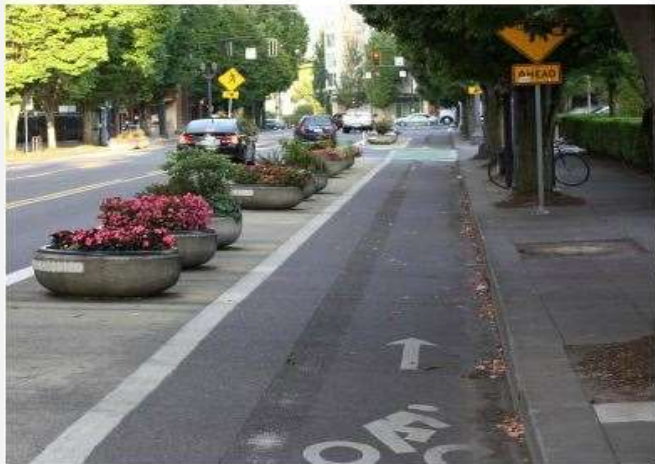
Exhibit 29. NE MULTNOMAH STREET LOOKING WEST (TOP), GRAPHIC SHOWING AERIAL VIEW (BOTTOM)
